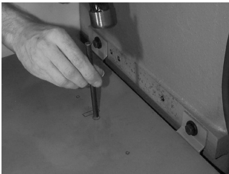
Figure 11-92 Center Punch Hole Locations for Drilling
